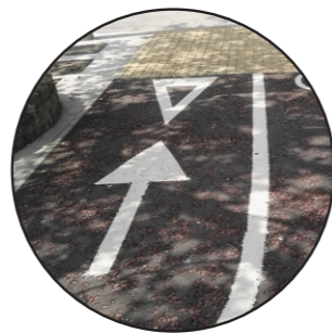
Cycleway Demarcation on Asphalt
