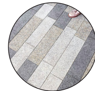
Threshold Pavement Precast Concrete Unit
