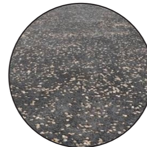
Asphalt with Chippings
