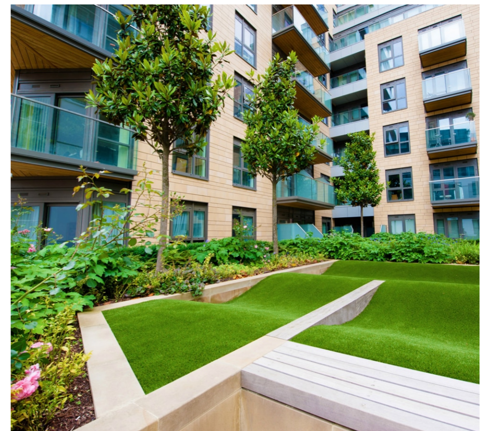
Intensive green roof - Dickens Yard apartments roof garden
