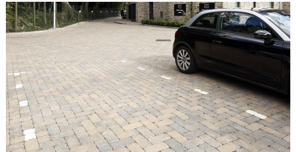
Shared surface and permeable pavement
