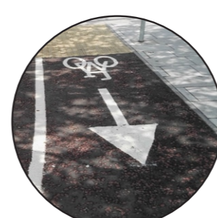
Cycleway Demarcation on Asphalt
