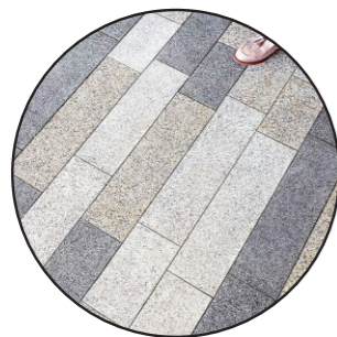
Threshold Pavement Precast Concrete Unit
