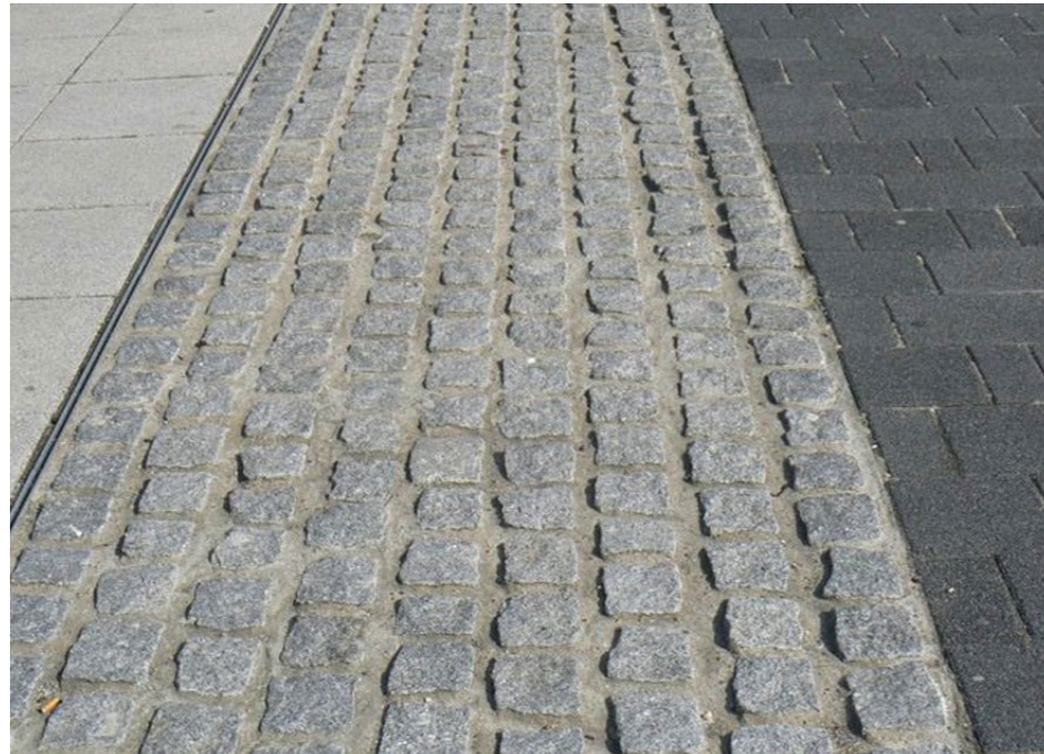
Feature setts and flagstones
