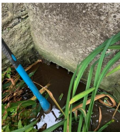
Photos 3.1 & 3.2. Existing drainage openings through the eastern perimeter wall. B1 on the right. B2 on the left (ref Fig 3.1)
