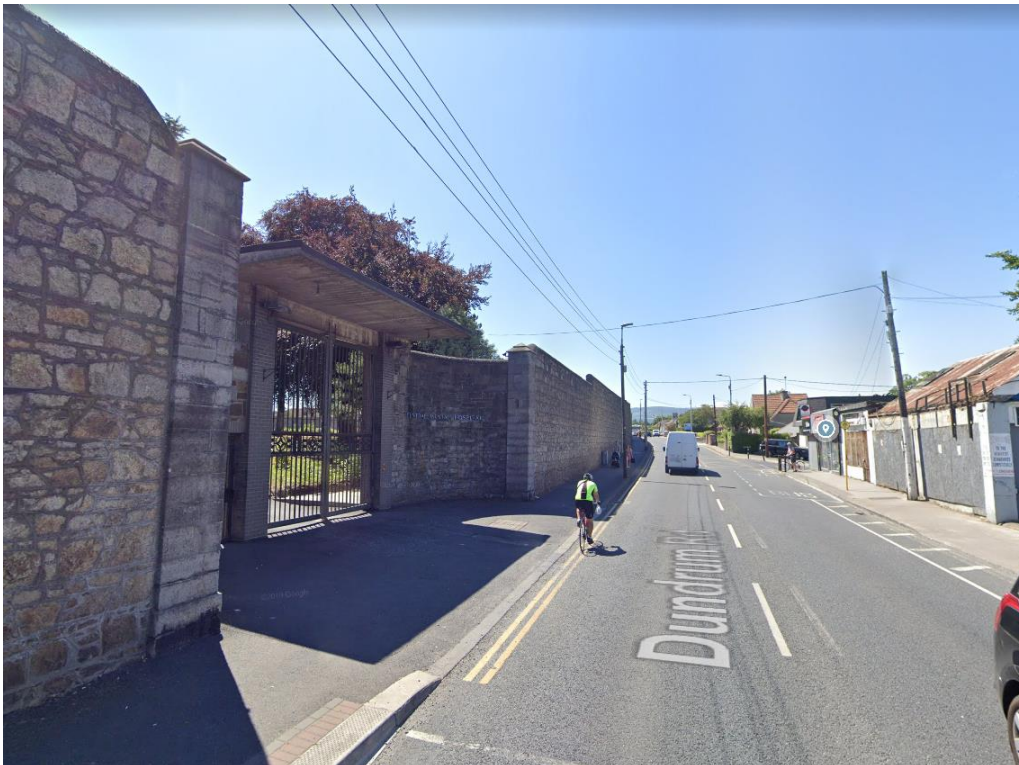
Photo 7.1 Existing access off the Dundrum Road R117 – Looking South
