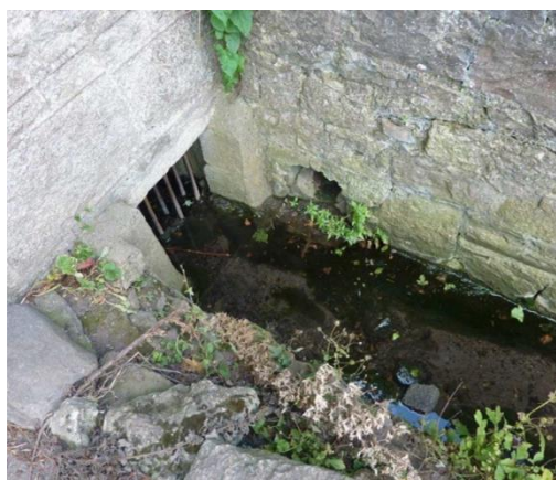
Photos 3.1 & 3.2. Existing drainage openings through the eastern perimeter wall. B1 on the right. B2 on the left (ref Fig 3.1)
